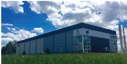
IPL Advancion Energy - 20 MW
